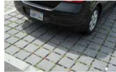
3 Stormwater is infiltrated through the use of permeable paving systems, landscape planters and other purposely located pervious surfaces.
